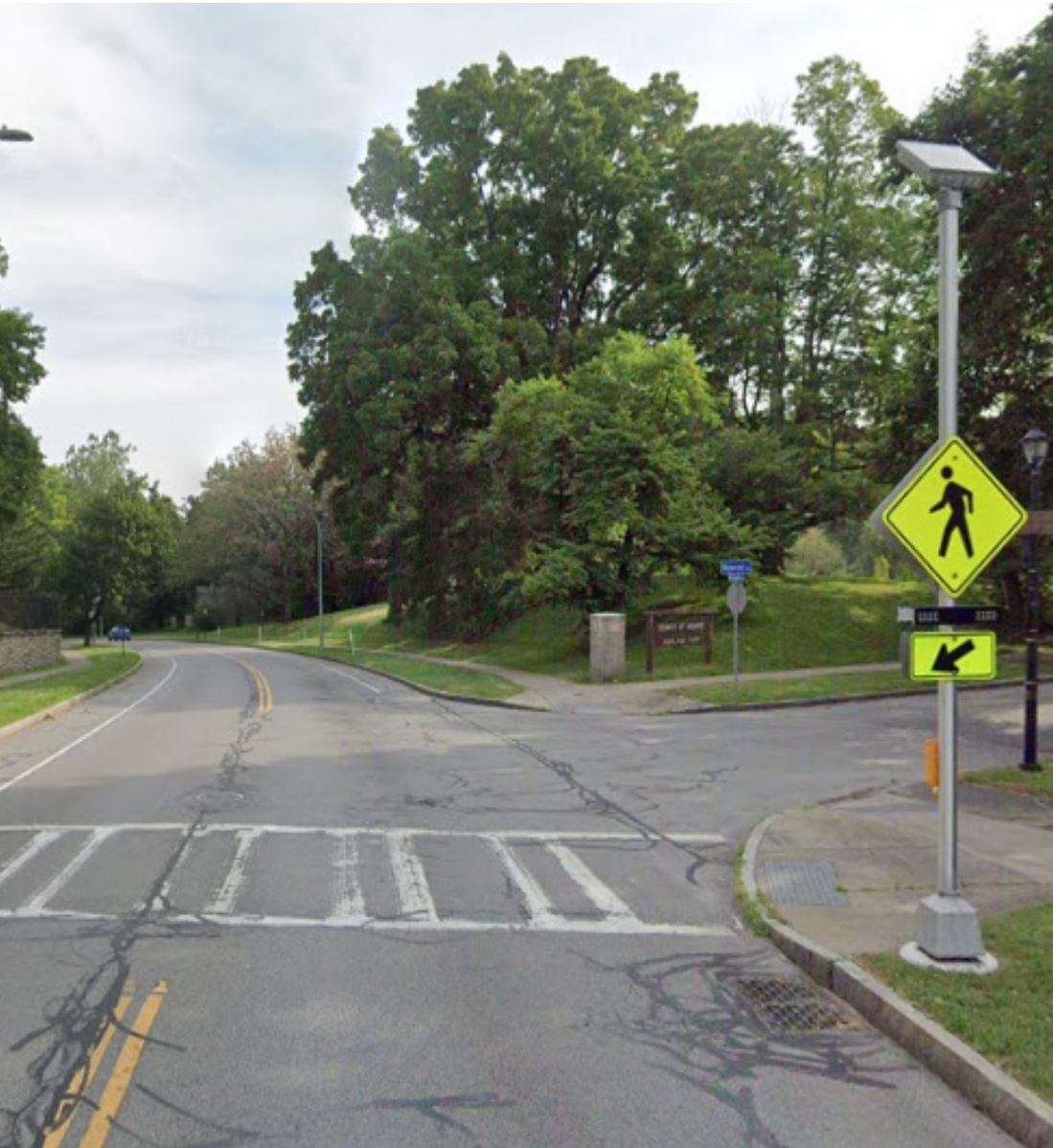
Rectangular Rapid Flashing Beacons (RRFB) at Mt Hope Ave and Reservoir Ave
