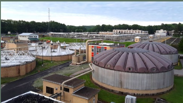
Monroe County Water Resource Recovery Facility
